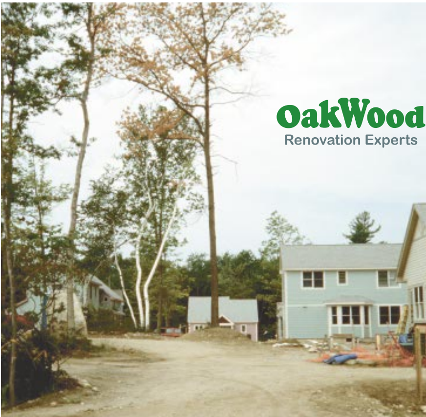
Figure 7. Lowering the grade around this oak has left it with practically no root system. The thin and discolored foliage shows that it's already dying. The inhabitants of the blue house at right might want to sleep in the basement on windy nights.
