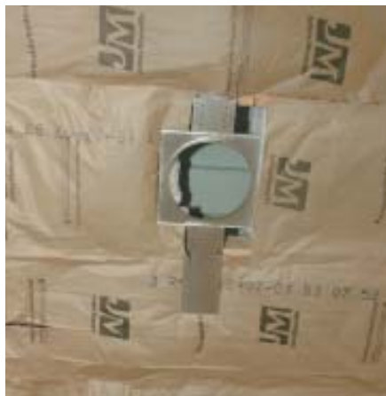
Figure 8. The rear speakers work equally well in the wall or ceiling. Everyone on site will have an opinion about where they look best, but check with the theater designer to find out where they'll sound best.
