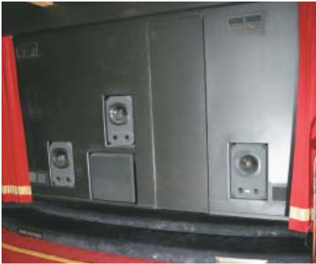
Figure 9. The front speakers in this theater project audio straight out through a sound-permeable viewing screen. In this photo, the screen has been retracted into the ceiling. The door and air intakes pass into the rack room behind the wall.
