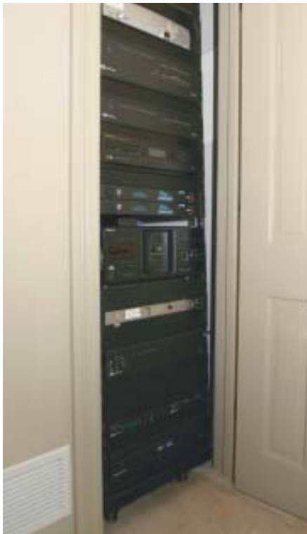
Figure 11. The theater in this house is part of a larger home automation system. All the electronic components are housed at a remote location in a closet or rack room.
