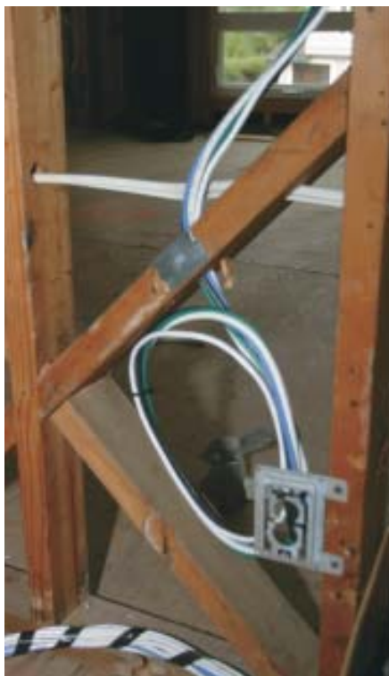
Figure 4. Ideally, A/V cable would never come within 24 inches of electrical wire. If they have to run parallel, keep these wires apart. If a cable has to cross an electrical wire, do it at a 90-degree angle as shown.
